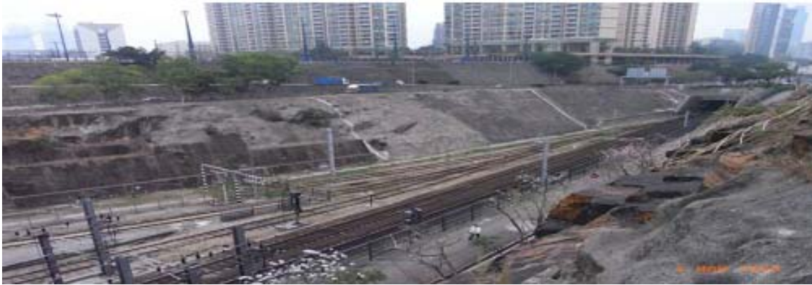
改善前 Before Improvement
